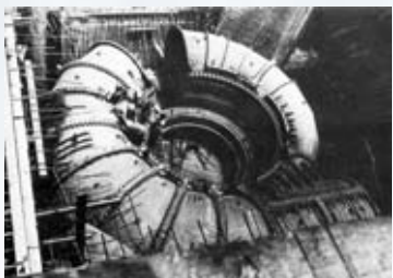
A 150,000 HP Francis waterwheel and casing being installed. The orders for these products generated a dramatic rise in Hitachi's exports.
