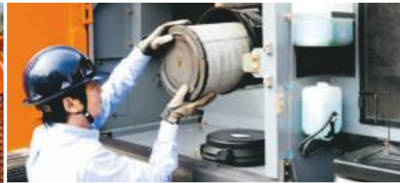
Ground level inspection made easy
